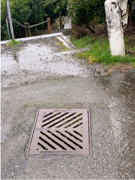
Catch Basin – Point E Top of Trail
