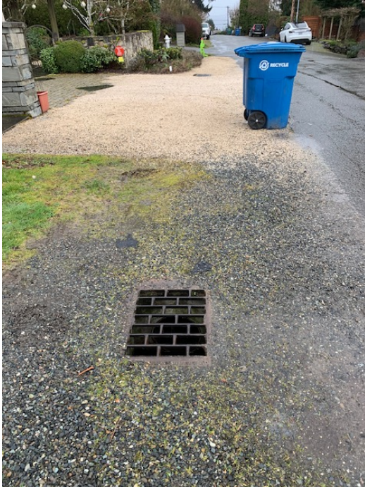
Catch Basin – At point B, Looking Downstream
