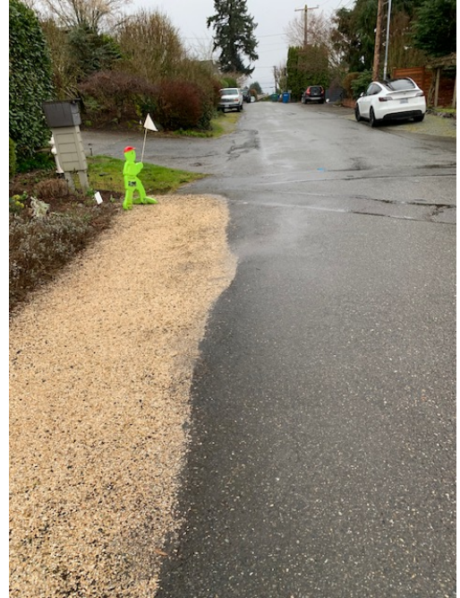
Looking Downstream from Catch Basin – At Point C
