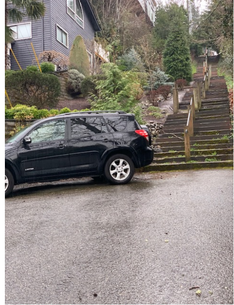
Catch Basin under Car at Point F at end of trail
