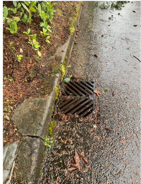
Catch Basin along Noth side of SE 32 nd Street, At Point J
