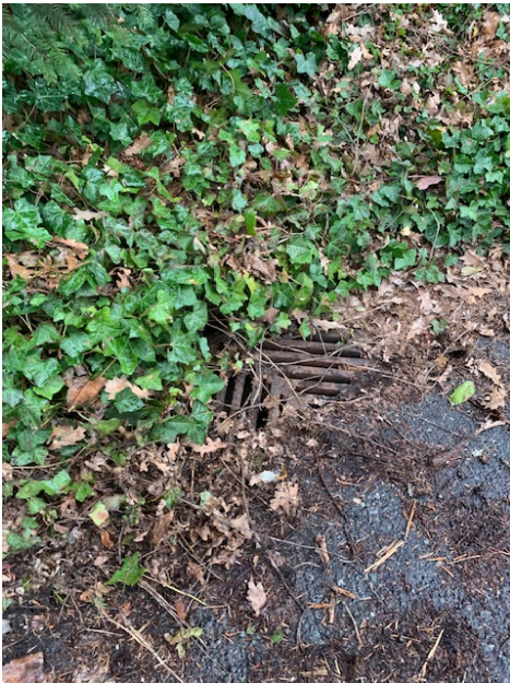
Catch Basin at South Side of SE 32 nd Street, At Point K
