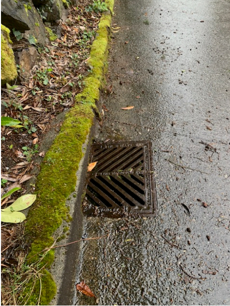
Catch Basin along South Side of SE 32 nd Street, Downstream of Point J
