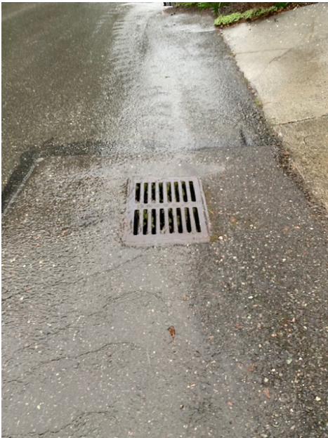
Catch Basin along Noth side of SE 32 nd Street, Downstream of Point H
